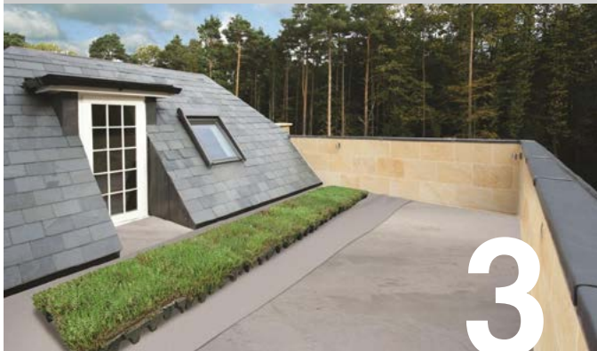
GrufeTile's are clipped together on the protection fleece
