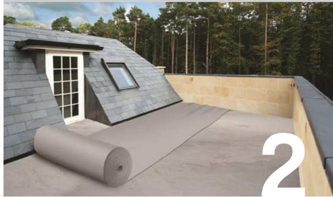
Protection fleece placed over your roof membrane
